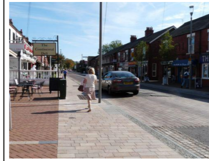
Flush surfaces encourage driver caution
